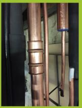
**Steve Gibbons from Ecotemp Environmental** welcomed the safety aspect of Zoom-Lock: "As we all know, hot works can be a pain and a fire hazard if you are in a tight space with brazing equipment, such as when you have a lot of pipes going into one big air conditioning box. ZoomLock is a much safer way of joining the pipes and saves time as well."
