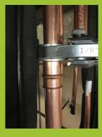
**Paul Dougan from Independent Cooling** explained how ZoomLock had already saved considerable time on a job. "We're installing HVAC into a new gym in a basement in London W1 where there is an existing VRF system which had leaks in both of the main pipes from the condenser, at high level in a very busy plant room.
